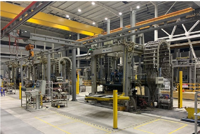
Casting line with furnace shuttle in the basement for the production of wheel carriers, structural parts as well as complete axle beams cast hollow
